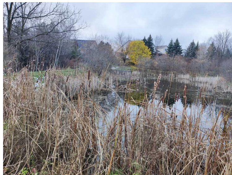
Photo of Hadati area stormwater management pond in Guelph
