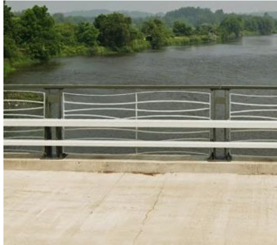
Fountain St., Cambridge. Image courtesy Google Earth
