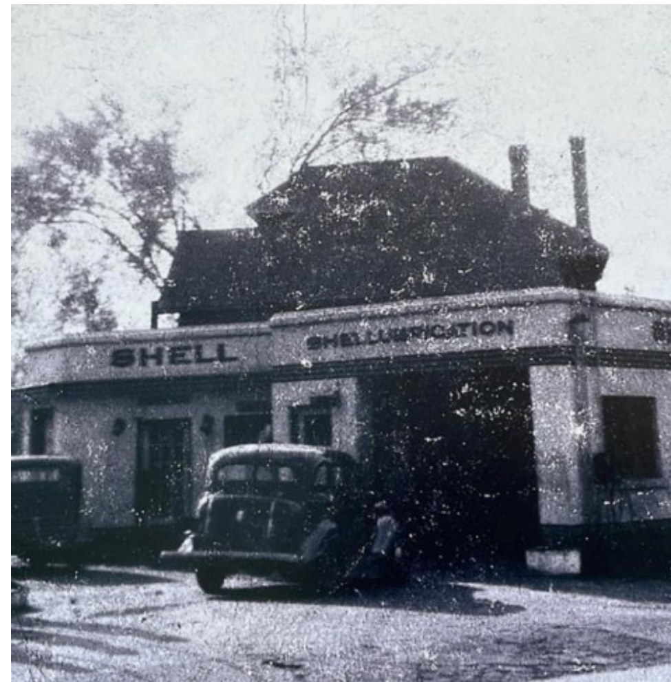
Figure 77: Bruno's Shell was located at 60 Ontario Street from the early 1940s to 1964, at the Ontario-Arthur-Manitoba Street intersection (GuelphToday, 2022)
