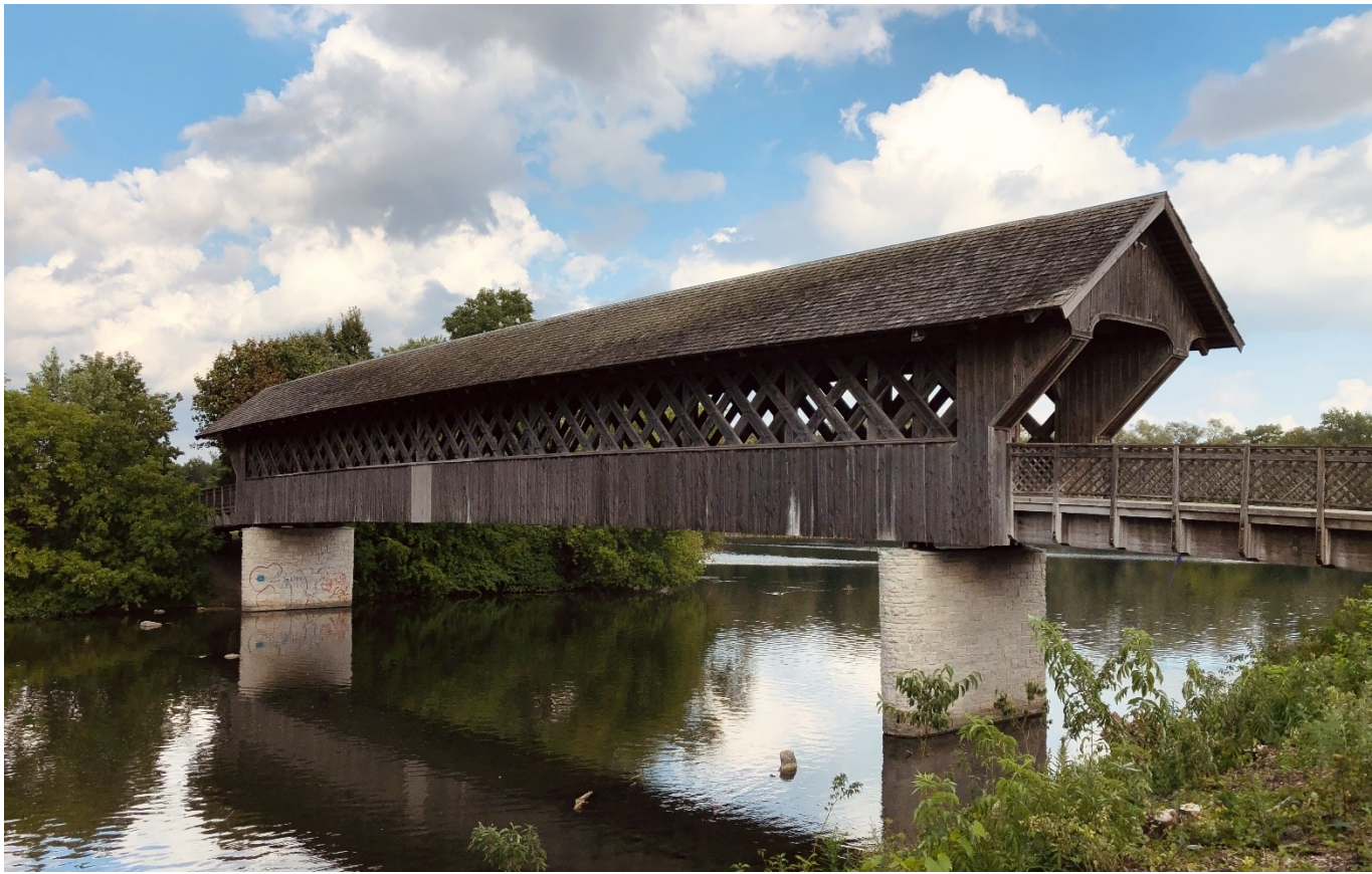
Figure 110: Covered pedestrian bridge crossing the Speed River (Photo courtesy of Jay Wall, O2 Planning and Design)
