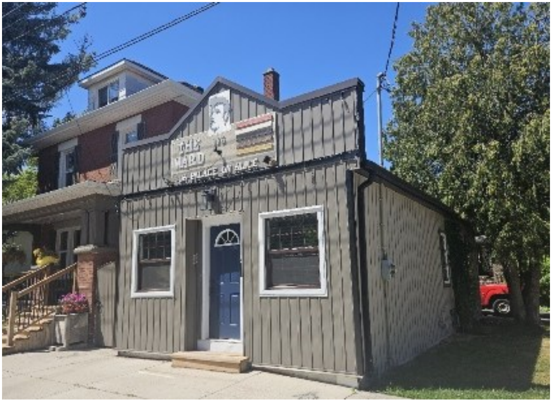
Figure 66: A false front façade is an architectural commercial pattern seen in the District (A.S.I., 2025)
