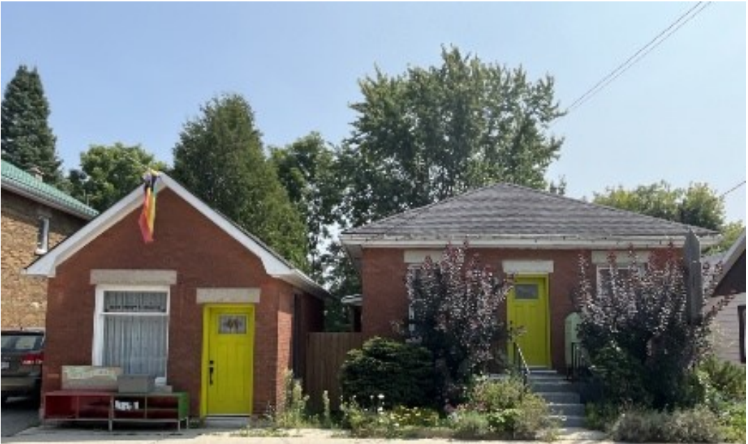
Figure 64: A small brick structure near or attached to a dwelling often indicates a historic shop (A.S.I., 2025)
