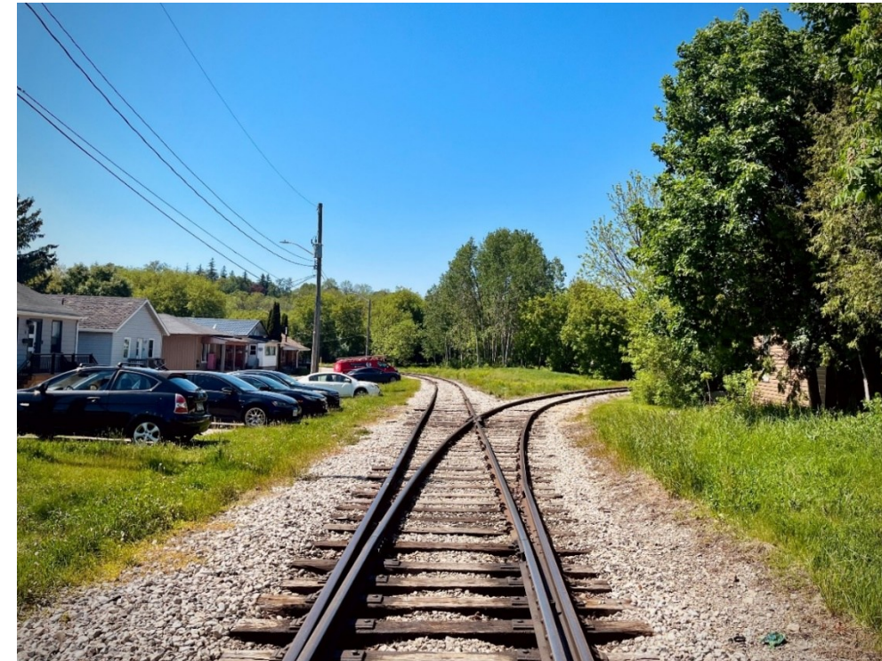
Figure 36: Railway tracks along Sackville Street (Jay Wall, O2 Planning and Design)
