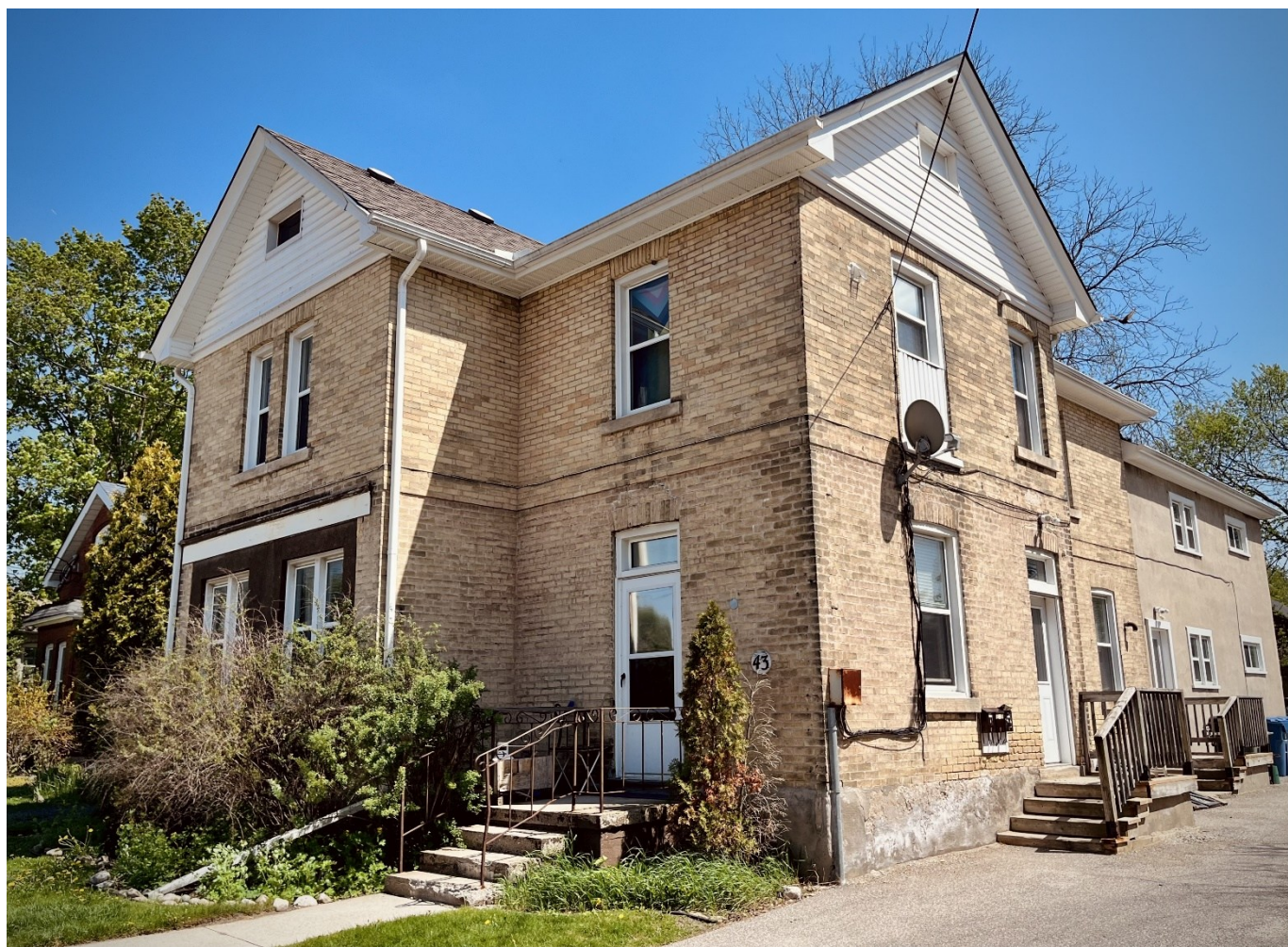
Figure 90: An existing example in the District with visible traces where a porch has been removed (Photo courtesy of Jay Wall, O2 Planning and Design)
