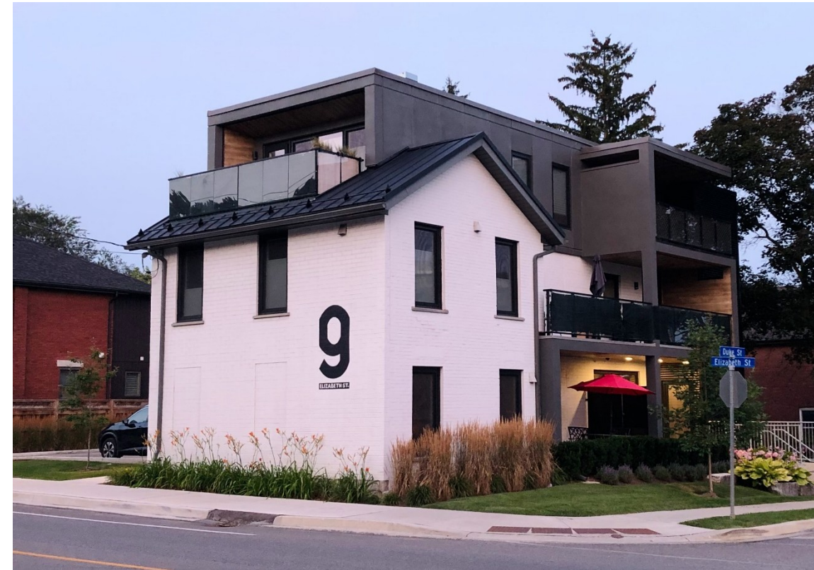
Figure 97: Example of an existing and permissible full-storey side yard addition in the District at 9 Elizabeth Street (Photo courtesy of Jay Wall, O2 Planning and Design)
