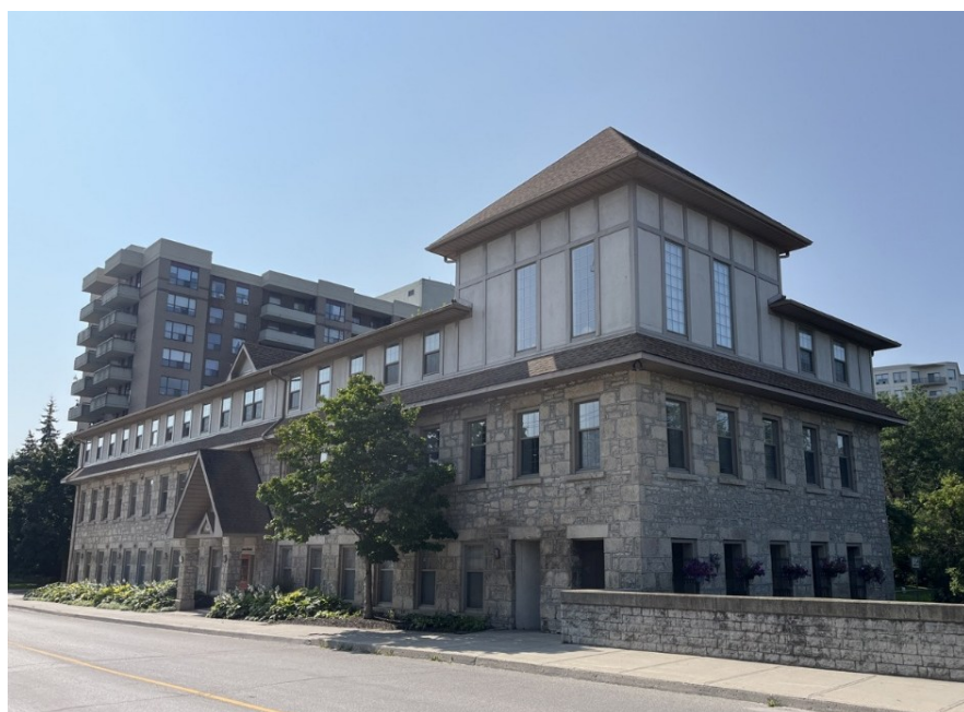
Figure 57: Previous factory at 83 Neeve Street, now a residential building (A.S.I., 2026)
