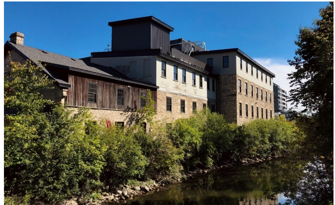
Figure 28: The former site of Allan's Mill shows the evolution of the industrial site along the Speed River, as pictured in 2025 (Photo courtesy of Jay Wall, O2 Planning and Design)
