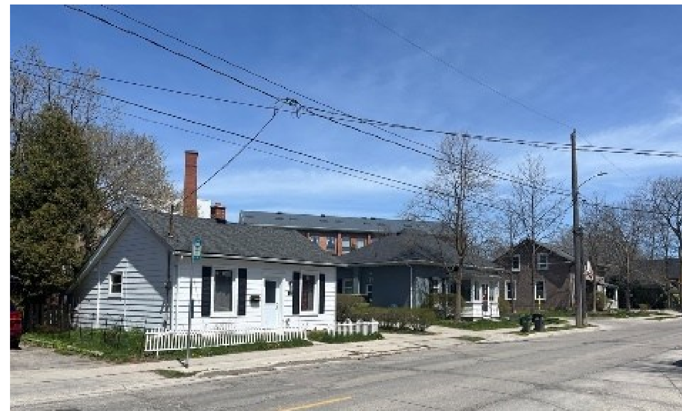
Figure 104 The small massing of one-storey Workers' Cottages creates a sense of space in the District even with small front setbacks (A.S.I., 2024)
