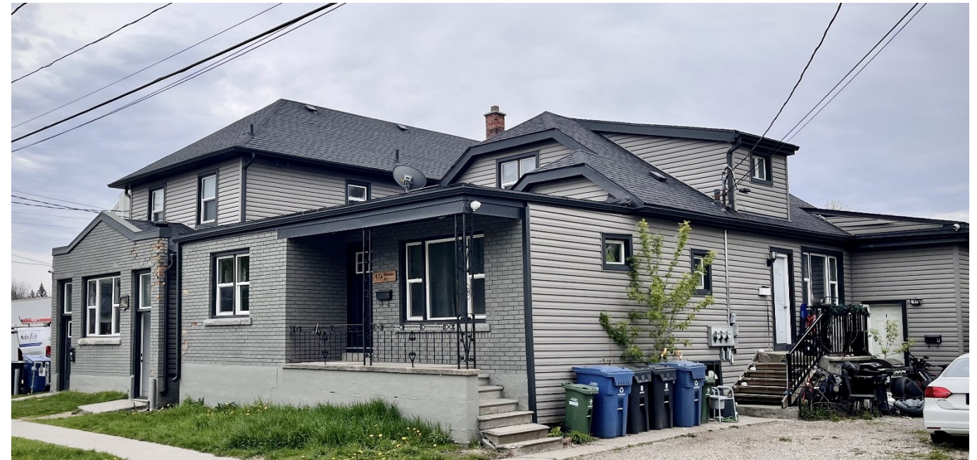
Figure 93: The primary buildings at 47-51 Huron Street have been retained through multiple additions (Jay Wall, O2 Planning and Design)
