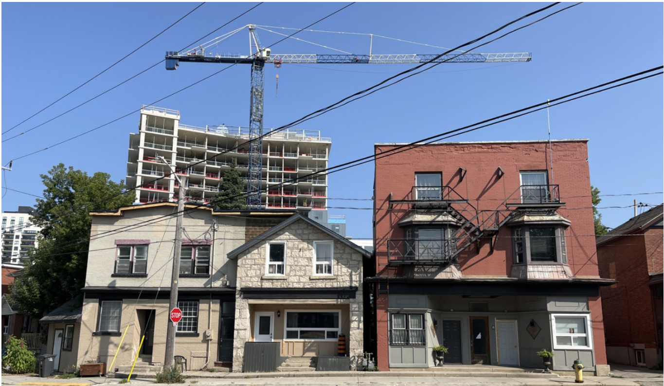
Figure 65: A series of adapted and purpose-built storefronts (now solely residential) along Ontario Street (A.S.I., 2024)
