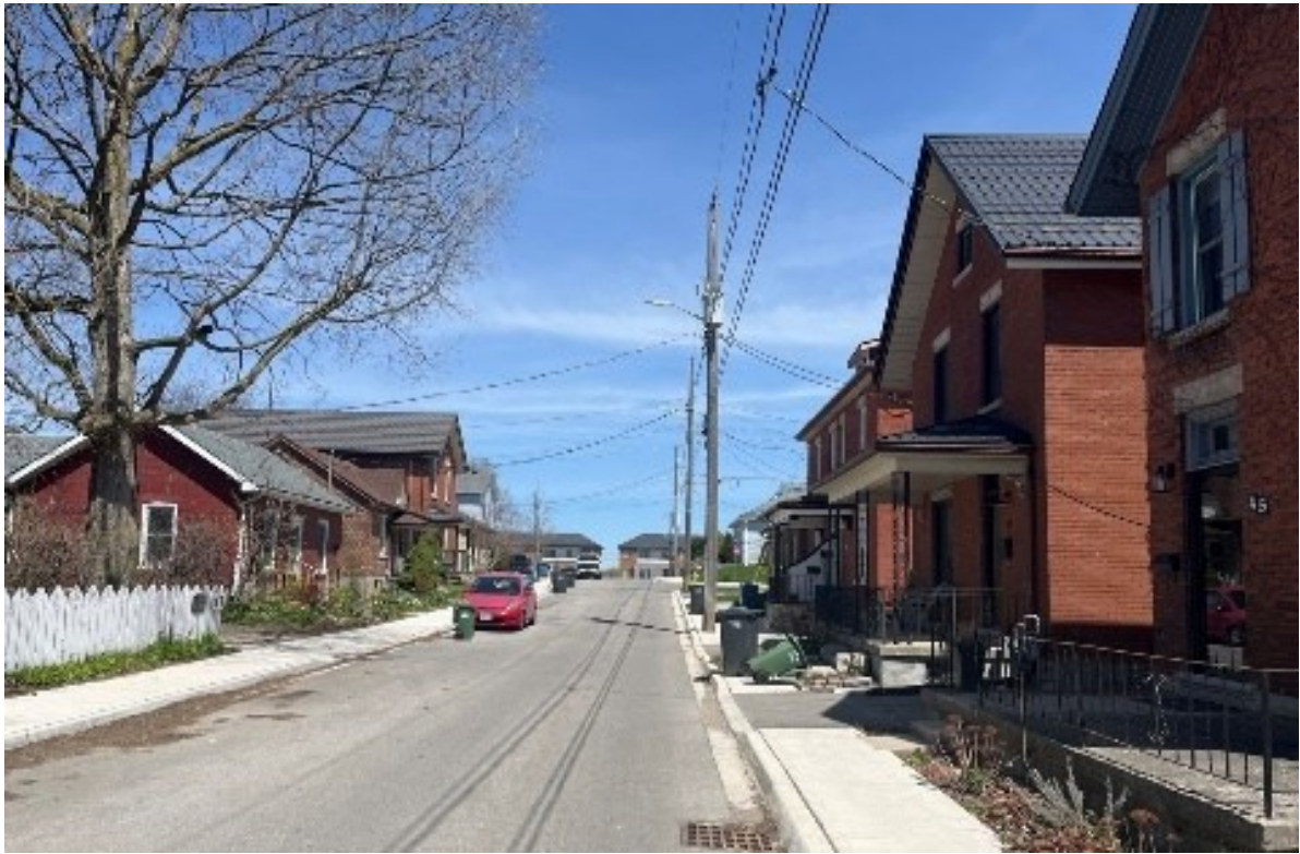
Figure 100: Typical massing in the District involves small-scale buildings and a mix of one- and two-storey heights within the same street (A.S.I., 2024)
