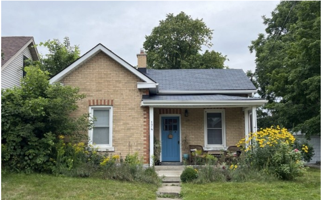
Figure 50: An early residence, constructed pre-1880 (A.S.I., 2026)
