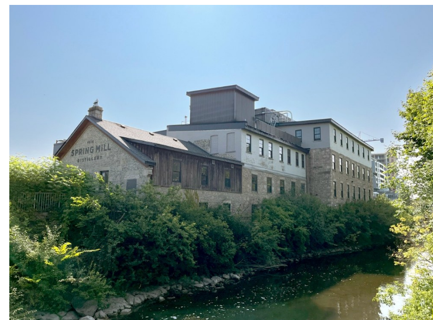
Figure 59: Today, 43 Arthur Street South is a multi-use building including a Distillery, a historic use at the site (A.S.I., 2026)
