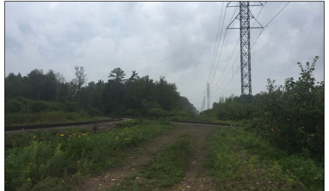
View of the GJR railway junction and Hydro One maintenance access road, looking north toward Marden Road
