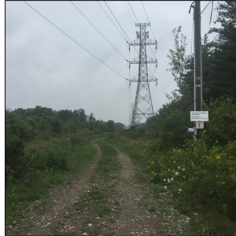
View of the Hydro One maintenance access road, looking north toward Marden Road
