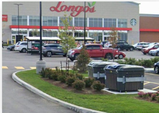
Photo 2: EarthBin Installation in a Commercial Setting in the City of Guelph
