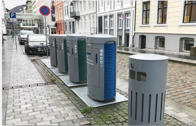
Photo 18: Underground Pneumatic System in the Medieval Center of the City of Bergen, Norway
