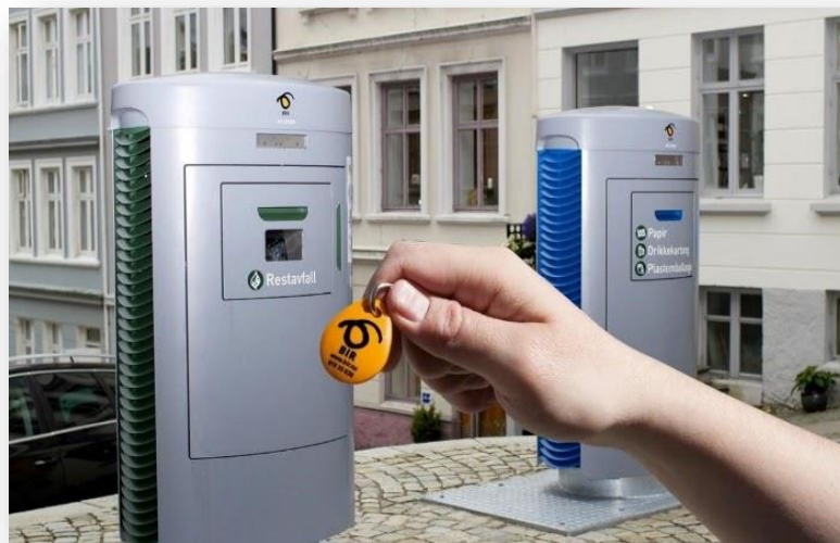
Photo 19: Underground Pneumatic System in the Medieval Center of the City of Bergen, Norway
