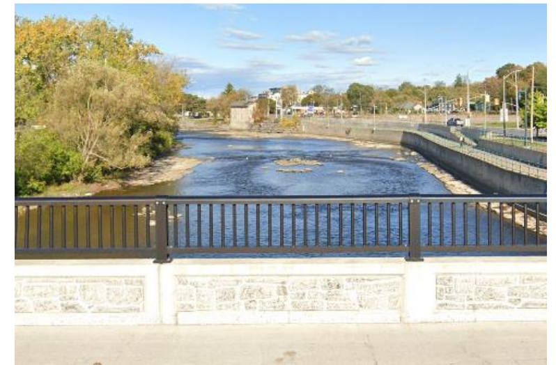
Sagonaska Bridge, Belleville. Image provided by Google Earth.
