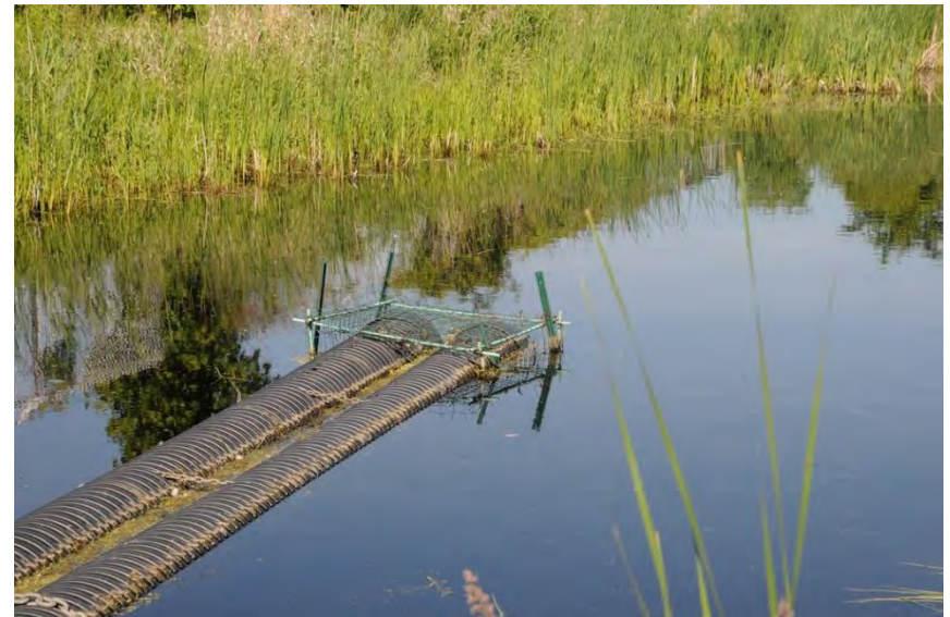
To the south of the tracks and approaching the hydro corridor is a stormwater pond for an adjacent industry with a beaver-proof outlet structure
