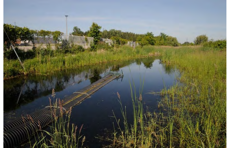
To the south of the tracks and approaching the hydro corridor is a stormwater pond for an adjacent industry with a beaver-proof outlet structure
