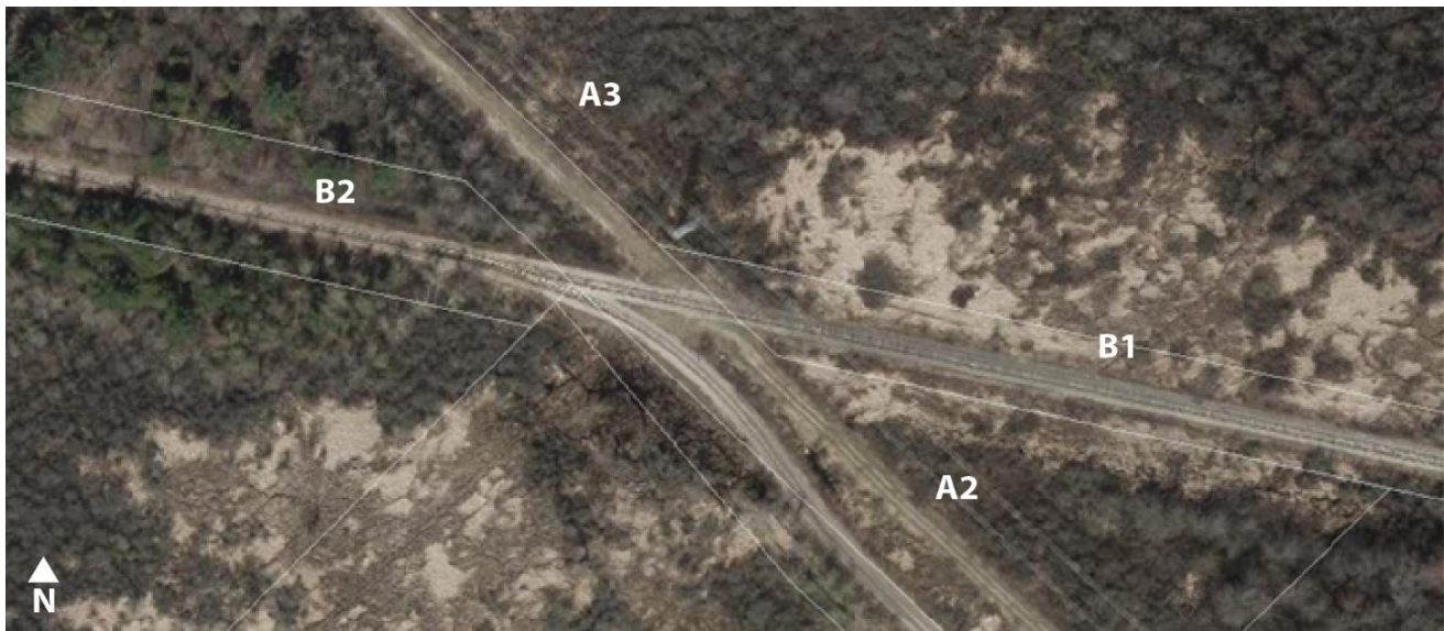
Figure 2 - Image showing the existing conditions at the GJR/Hydro Corridor junction
