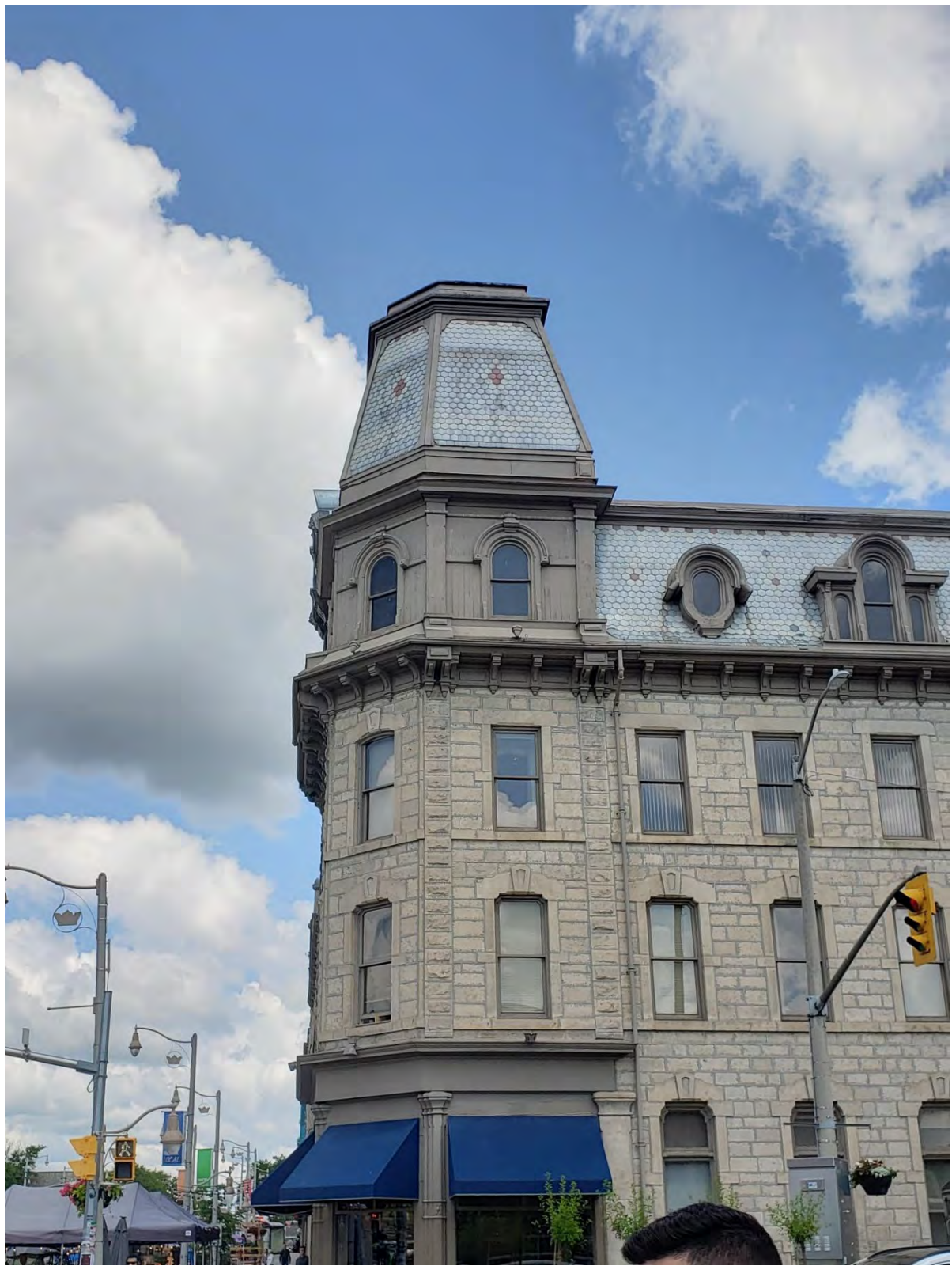
Figure 21: Decorative limestone work on the Sovereign Apartments on Macdonell Street (A.S.I., 2023).
