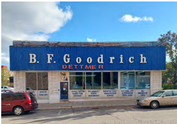
Figure 29: Dettmer Tire building with current cladding (A.S.I. 2023).
