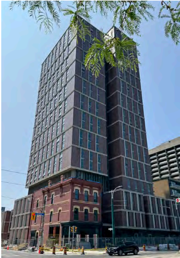
Figure 38: Example of a tall building addition to a heritage building employing, a step back, distinct massing and materials between the existing and new structures. Address: 700 Spadina Avenue, Toronto (Urban Toronto Database).
