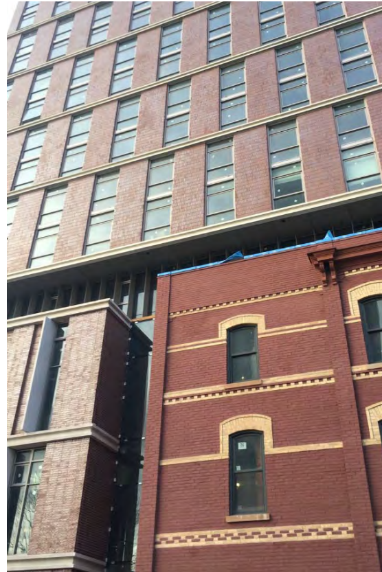
Figure 39: Detail of 700 Spadina Avenue, Toronto illustrating compatible materials (existing and new brick) separated by a physically articulated gap in a distinct material (glass) (Urban Toronto Database).
