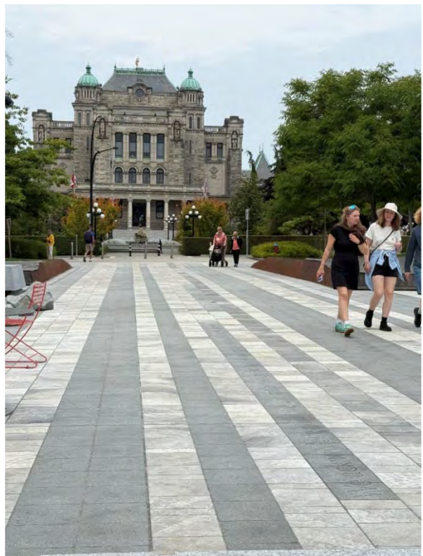
Figure 53: More accessible pavers at Capital Park in Victoria, British Columbia. The surface is lightly textured, low-glare, and the pattern is not visually overwhelming. The blocks are tightly jointed and define separate spaces for circulation and furnishings (Mark Steele, 2025).
